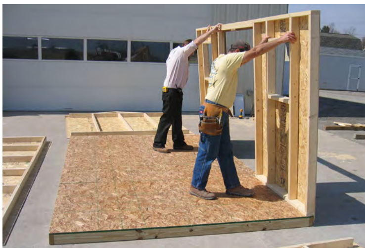
42. Now install the first wall, standing it up on the floor.
