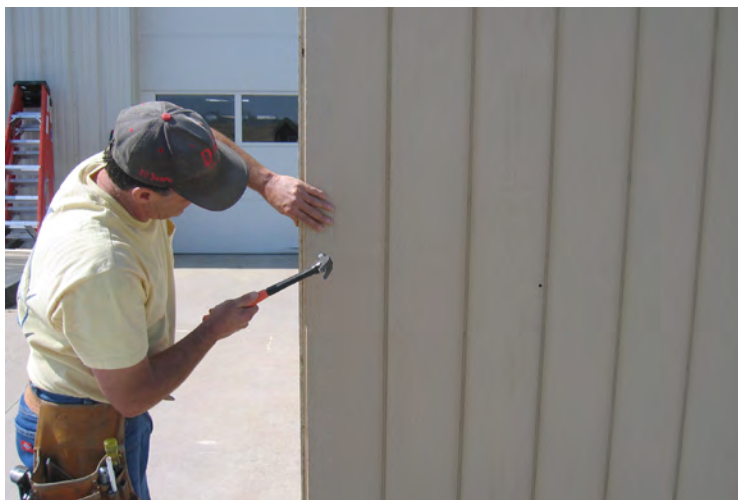
52. Nail the corners every 6" to 8" with 2" nails.
