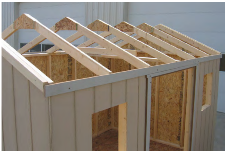
64. Continue installing the trim as shown.
