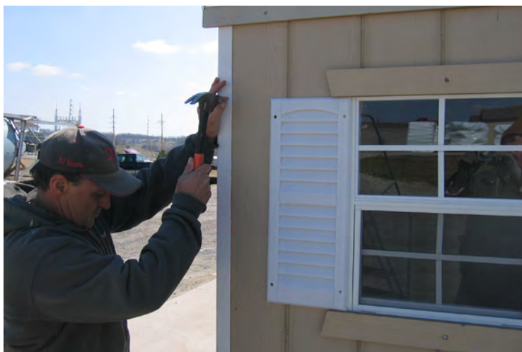
96. Locate the aluminum corner trim. Fasten the trim onto all four corners of the building with white finish nails.
