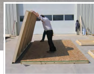
26. Lay wall to the side as shown.
