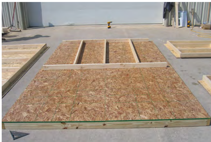
27. Using the wall layout diagram sheet, locate the wall plates and studs as shown.
