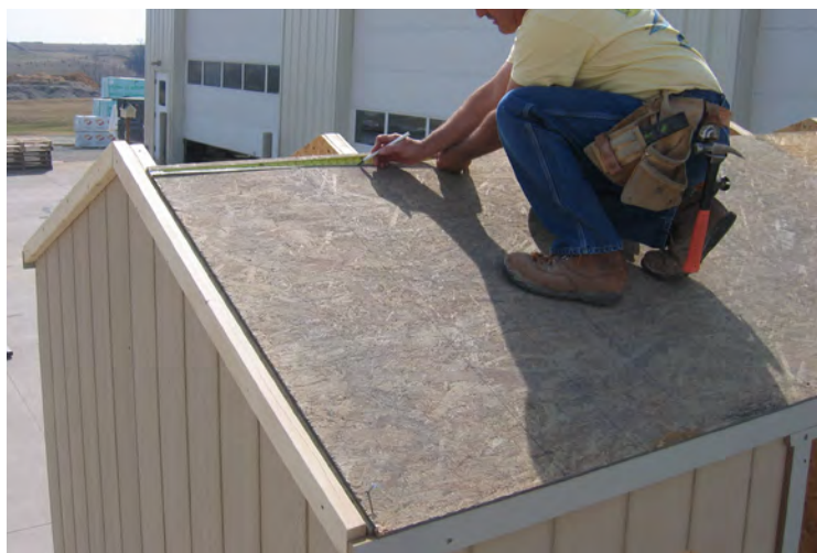
67. Make sure the trusses are 24" on center before fastening sheeting.
