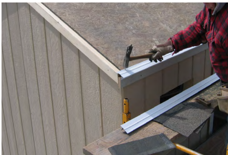
68. Next install the drip edge as shown (drip edge not included - see kit packing list for amount of drip edge you will need to purchase).
