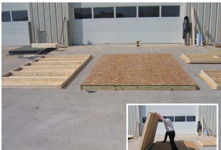
26. Lay wall to the side as shown.
