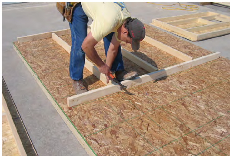
28. Secure with 3" nails as shown.
