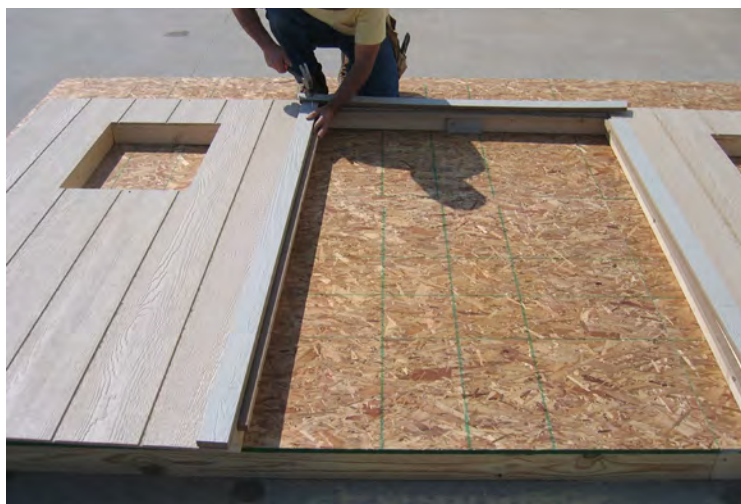
19. Install the 2 3/4" trim around the door. Secure the trim with 2" nails, staying at least 1 1/4" in from the inside edge, so they do not interfere with the hinge screws later.
