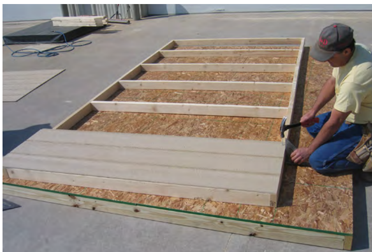
24. Continue installing, keeping the top-side flush.
