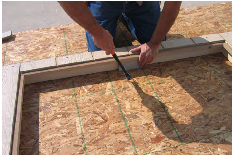
18. Install the trim block in the center of the header and secure with 2" nails.
