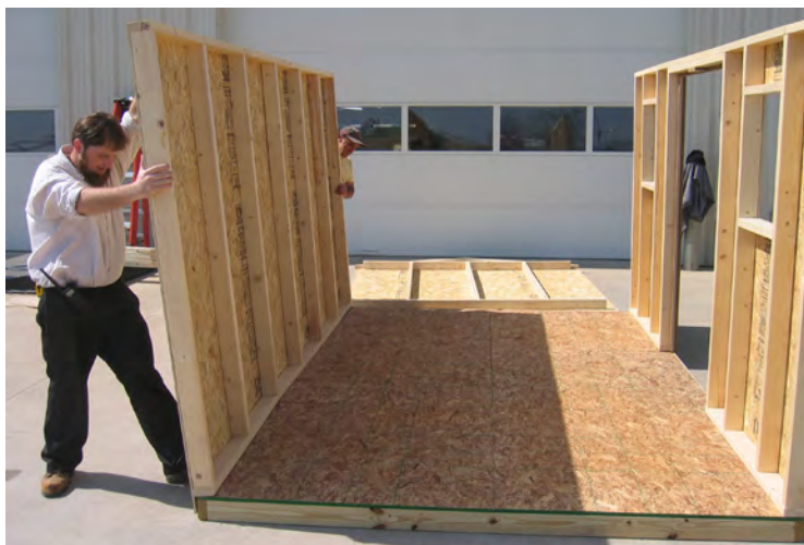
46. Continue with walls as shown.
