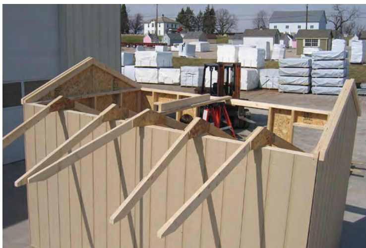
60. Next hang trusses on the walls as shown.
