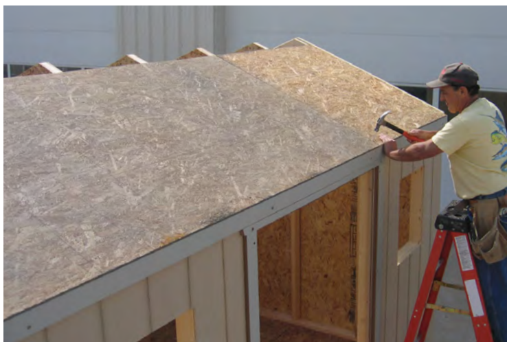
66. Continue with the roof sheathing.
