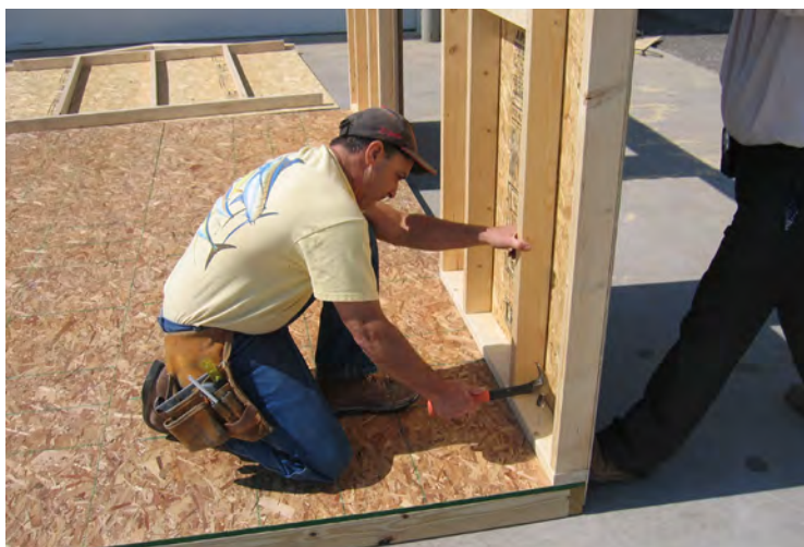
44. Fasten with 3" nails 16" on center.
