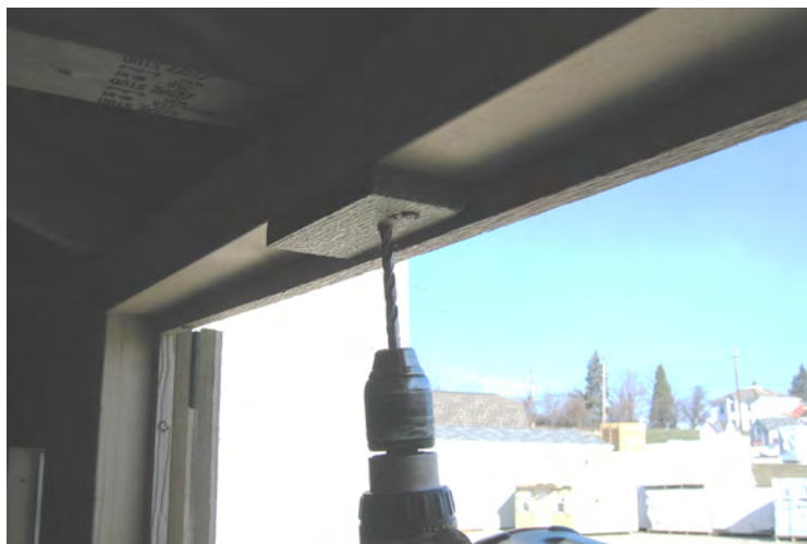
93. Drill a 5/16" hole for the barrel bolt.
