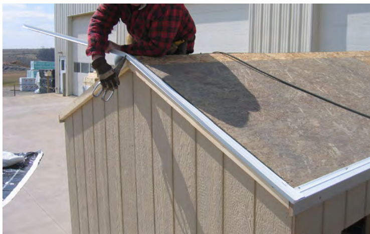
70. Use the tin snips to cut drip edge so it will bend.
