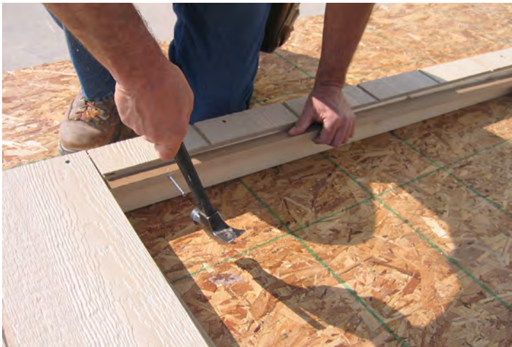
17. Next install door stops as shown. Keep flush with the top of 2x4 (not the Smartside) and secure with 2" nails.
