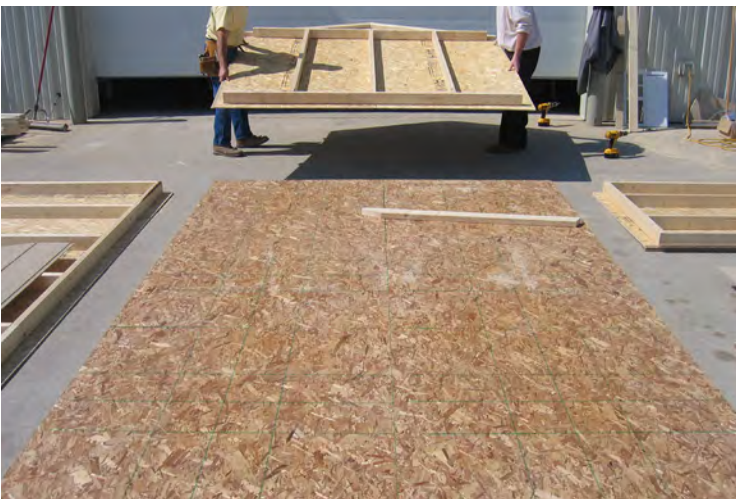
35. Lay wall to the side as shown.
