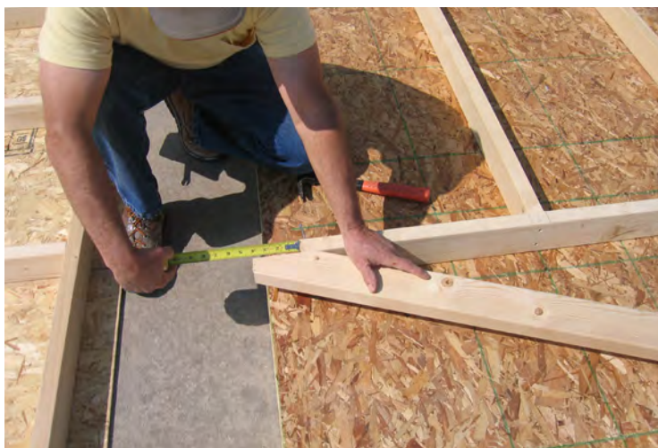
30. Measure out 3 7/8" from the edge of the top plate to the end of the truss.
