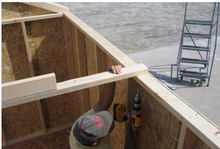
58. Attach the temporary braces to the wall with 2 1/2" screws.
