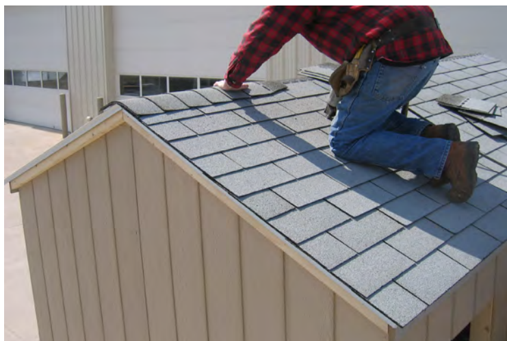
77. Continue placing the ridge cap, as shown.
