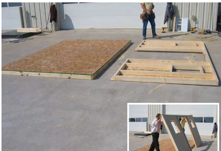
20. Lay wall to side as shown.
