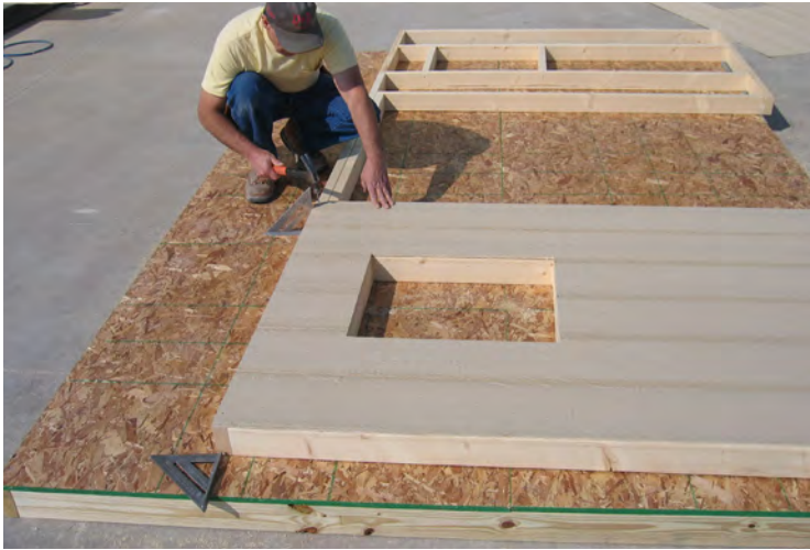
13. Next make sure the top of the siding is flush with 2x4 studs.
