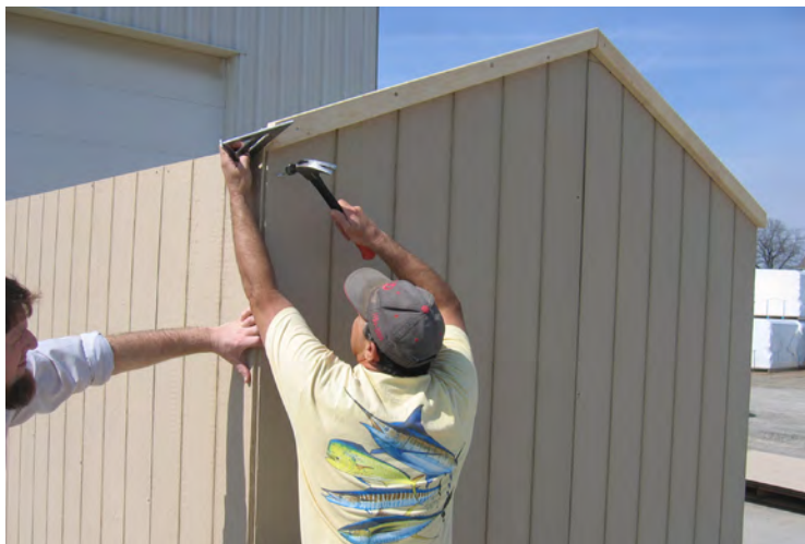
48. Fasten outside corner as shown with 2" nails.
