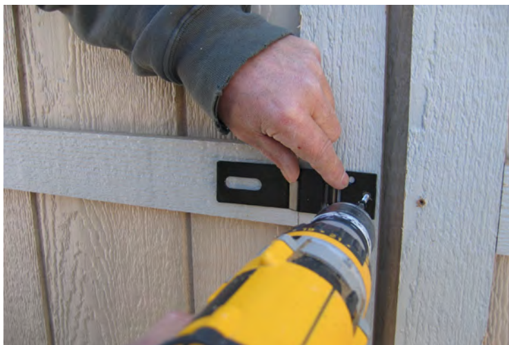
94. Locate the latch. Install half of the latch, as pictured, on one of the doors, with 1 1/4" screws.
