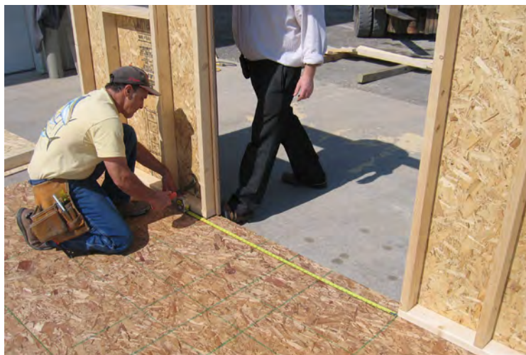
45. For the doorway, make sure you have 48" or 60" (depending on the building width) in between the door opening, 48" on 8' wide buildings and 60" on 10' and wider buildings.
