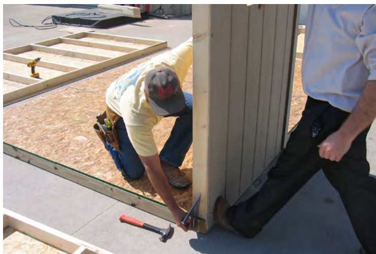
43. Make sure the wall is flush on the end and put pressure on the outside as shown, fasten with 3" nails.
