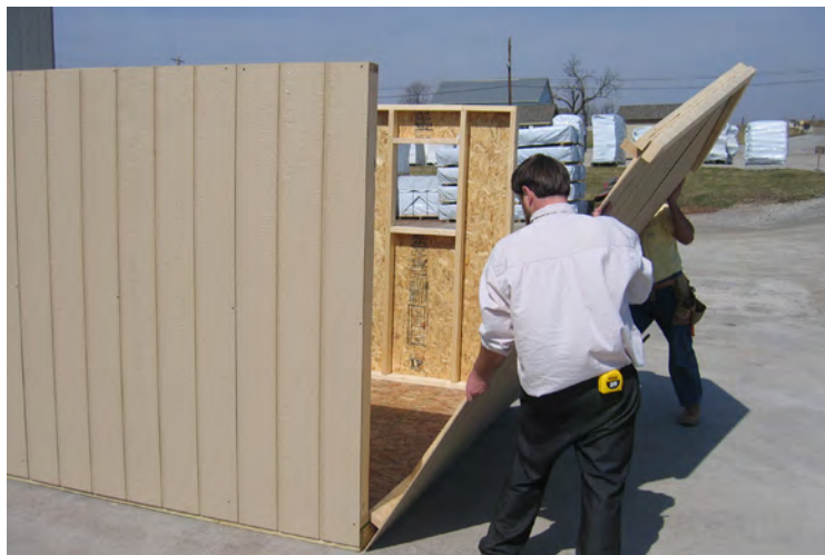
47. Continue with walls as shown.
