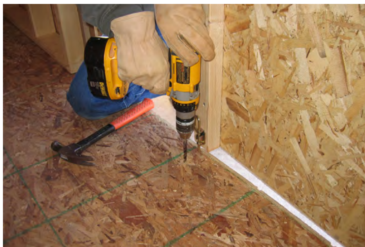
91. Drill a 5/16" hole as shown.
