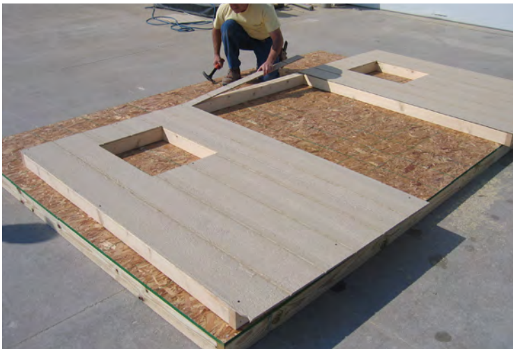
15. Continuing with Smartside siding installation, place the header piece into place.
