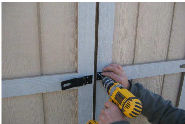
95. Line up and install the other half of the latch on the opposite door.
