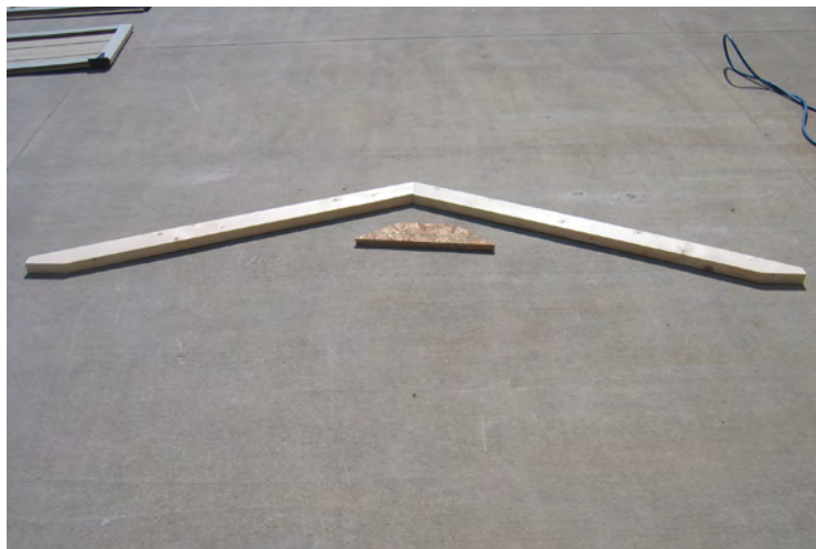
53. Next locate the truss parts.
