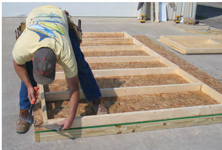
21. Using the WALL LAYOUT DIAGRAM SHEET build the next wall.
