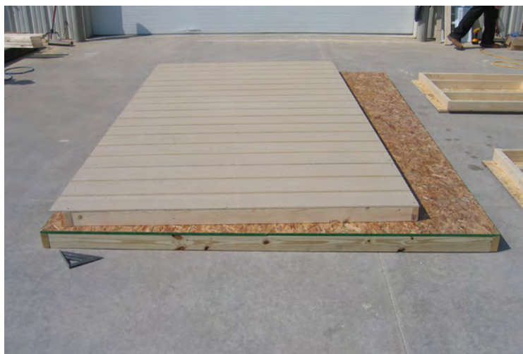
25. Continue with Smartside and fasten with 2" nails every 6 to 8 inches.
