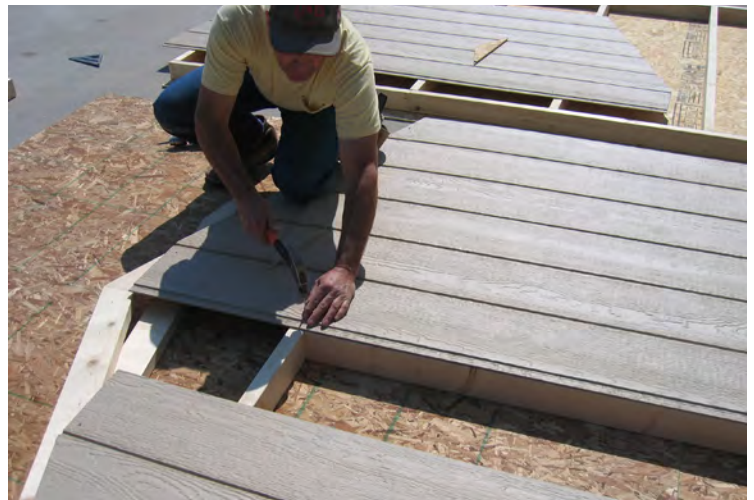
34. Secure with 2" nails every 6" to 8" on center.
