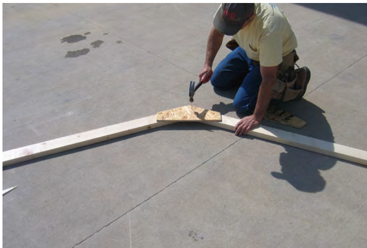
54. Install the truss gussets as shown and secure with 2" nails.
