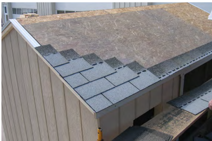
74. Install shingles in a staggered fashion.
