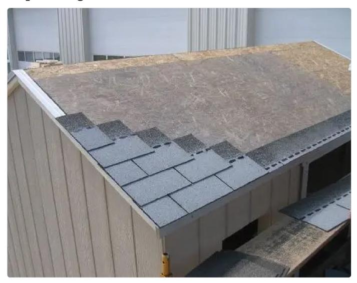
Install drip edge and roof shingles (not included, available at local hardware store).
