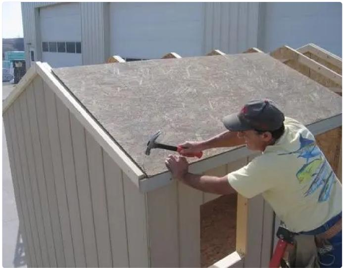
Install the trusses and sheathing.
