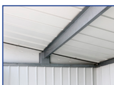
Strong Steel Roof Truss
