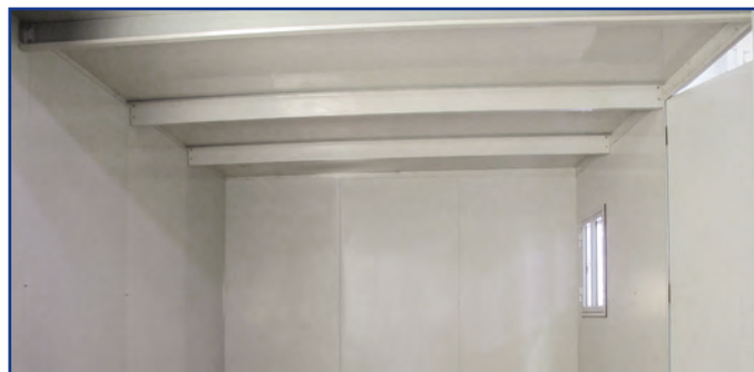
Building reinforced with metal columns and beams
