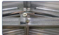
Front Door Cable Pulley System
